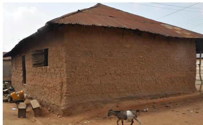
Figure 1. A typical mud-built house.
